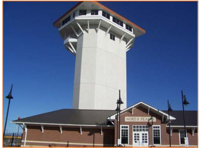
Tower, North Platte Railroad Yard
